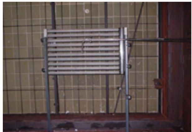
**4. Supplemental AIG assembly** installed at Clearwater Cogen
