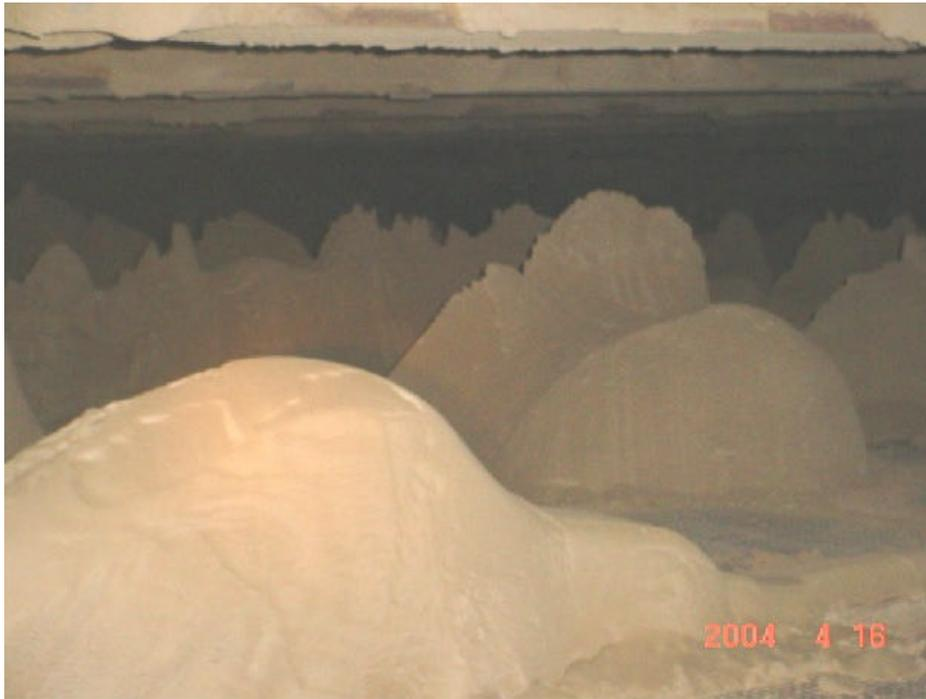
**Figure 8b.** Deposits of Ash on Turning Vanes
